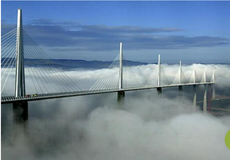
The Viaduc de Millau is the longest cable-stayed bridge in the world (2460 m). About 19,000 tons of steel were used for concrete reinforcement, 5,000 t were used for the cables and stays. Source: http://www.abelard.org/france/viaduct-demillau.php#viaduc ).
