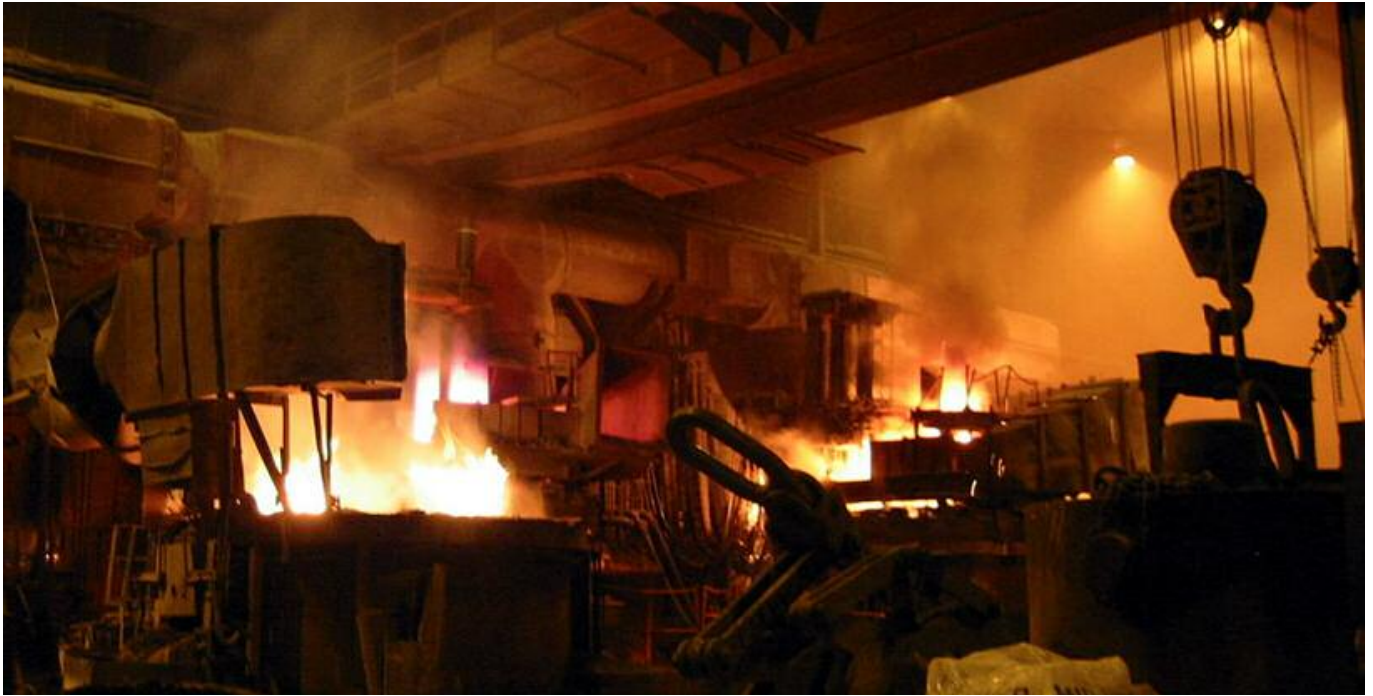
Figure 4: Steel mill with two electric arc furnaces; each furnace consists of a refractory lined hearth, in which the feedstock is molten down using one or more graphite electrodes which enter the furnace through the refractory-lined roof. EAFs are the heart of a special steel production. To follow charge formation and meltdown is very spectacular but dangerous; melt capacity is commonly between 50 to 80 t, but can go up to 300 t. Tungsten is added to the furnace charge either as tungsten scrap or in the form of ferrotungsten. http://en.wikipedia.org/wiki/Electric_arc_furnace
