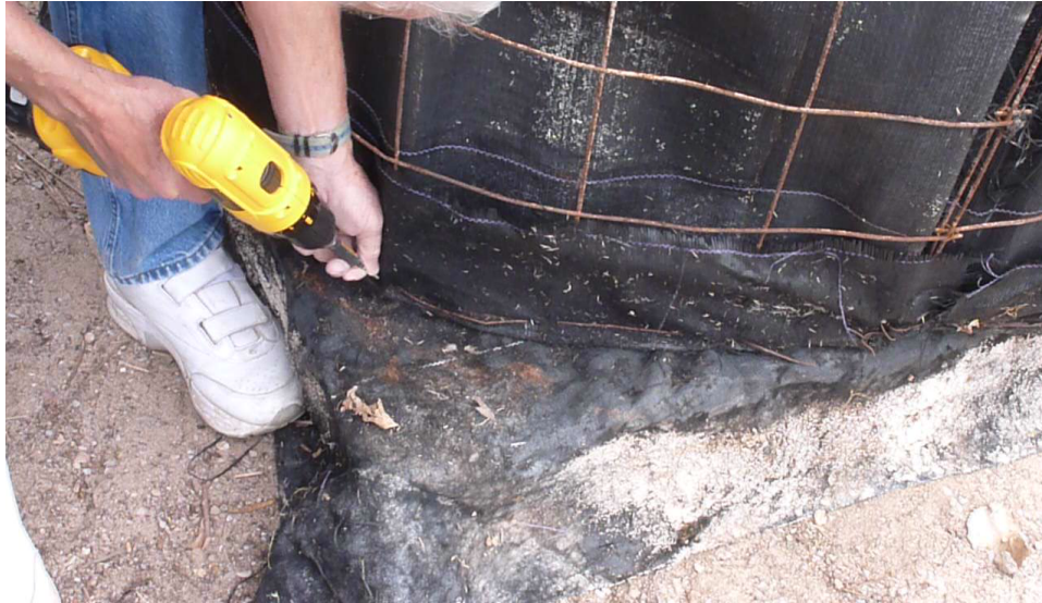
Figure 5. Screwing the Base of the Cage to the Pallet
