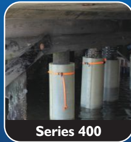
Timber Pile Structural Repair
