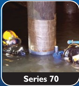
Timber Pile Protection
