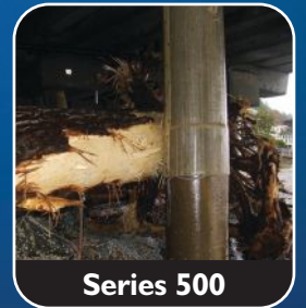
Epoxy Grout Encapsulation System
