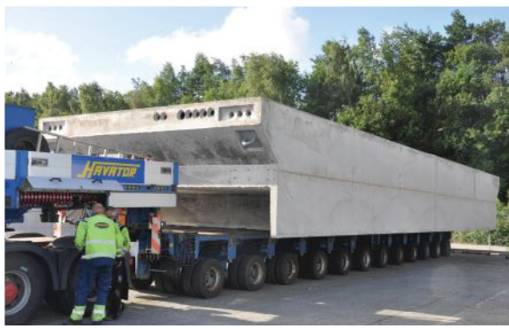
20' Wide Floating Breakwater
