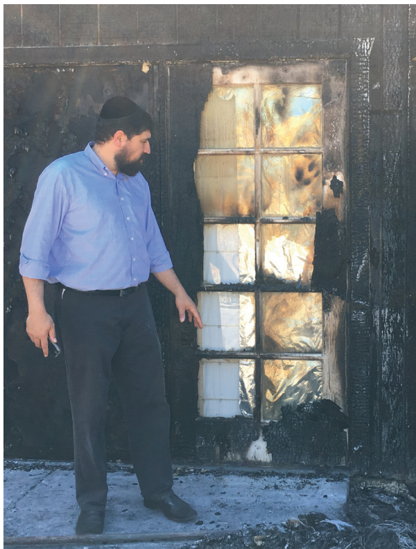
Rabbi Raleigh Resnick surveying the damage on Aug. 12. (Photos/Gabe Stutman)
