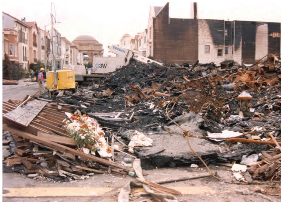
Earthquake damage in the Marina District (Photo/Wikimedia Commons)
