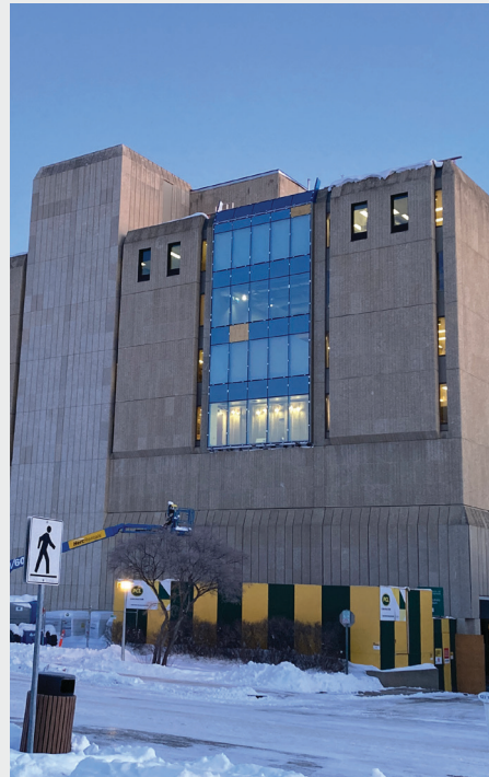
The 'waterfall' window during installation.
